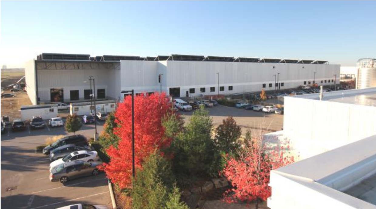
Systems Center in early November 2014; existing building in foreground
